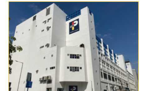
PARKnShop Frozen Warehouse
